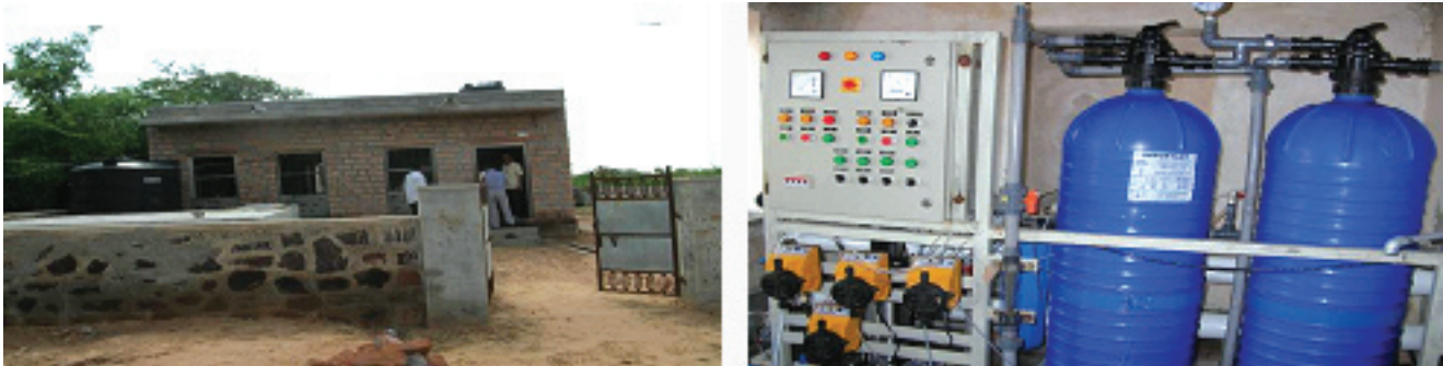
RO Plant in Pachpadra, Barmer district
