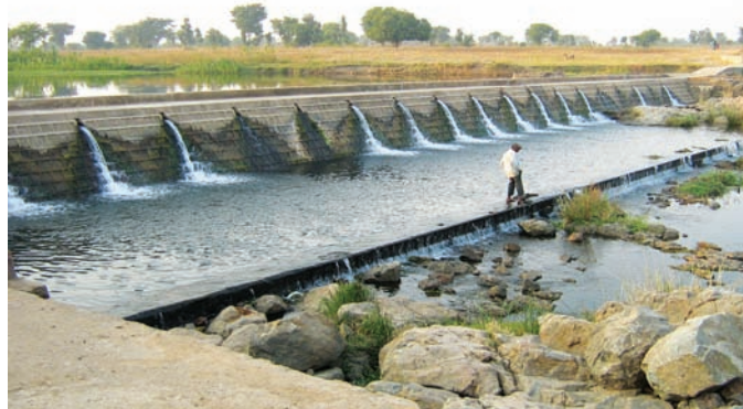
Water Harvesting Structure
