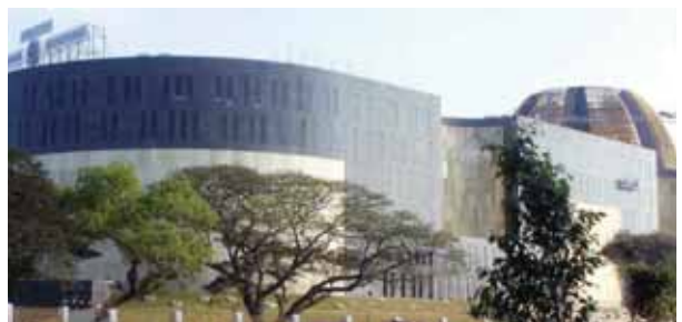
CII-Sohrabji Godrej Green Business Centre, Hyderabad, India's First Platinum rated LEED Green Building (top) Tamil Nadu Legislative Assembly Building, Chennai, World's First Green Legislative Assembly
