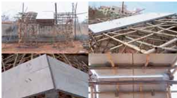
Experimental structure at International Institute of Information Technology, Hyderabad
