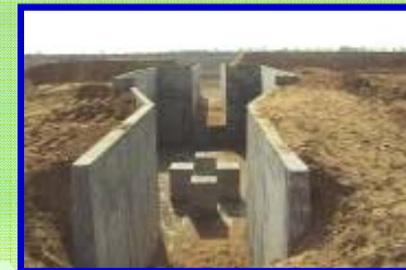
Desilting Chamber
