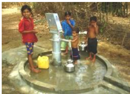
Fig: Installed Hand Pump
