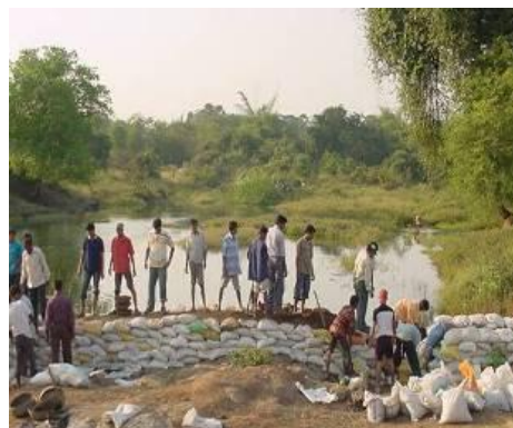
Fig: Check Dam under Construction
