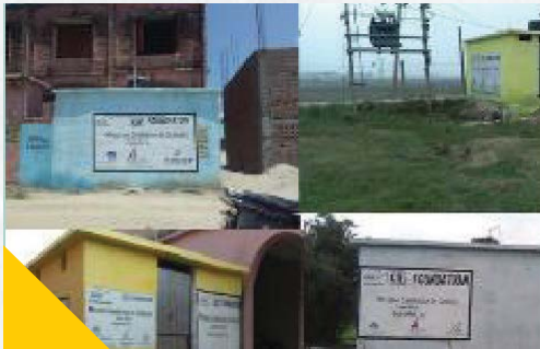
School Toilet Blocks Constructed in Bihar
