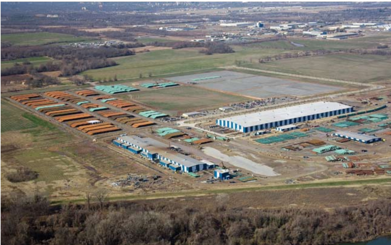
Welspun Manufacturing Facility, Little Rock, Arkansas
