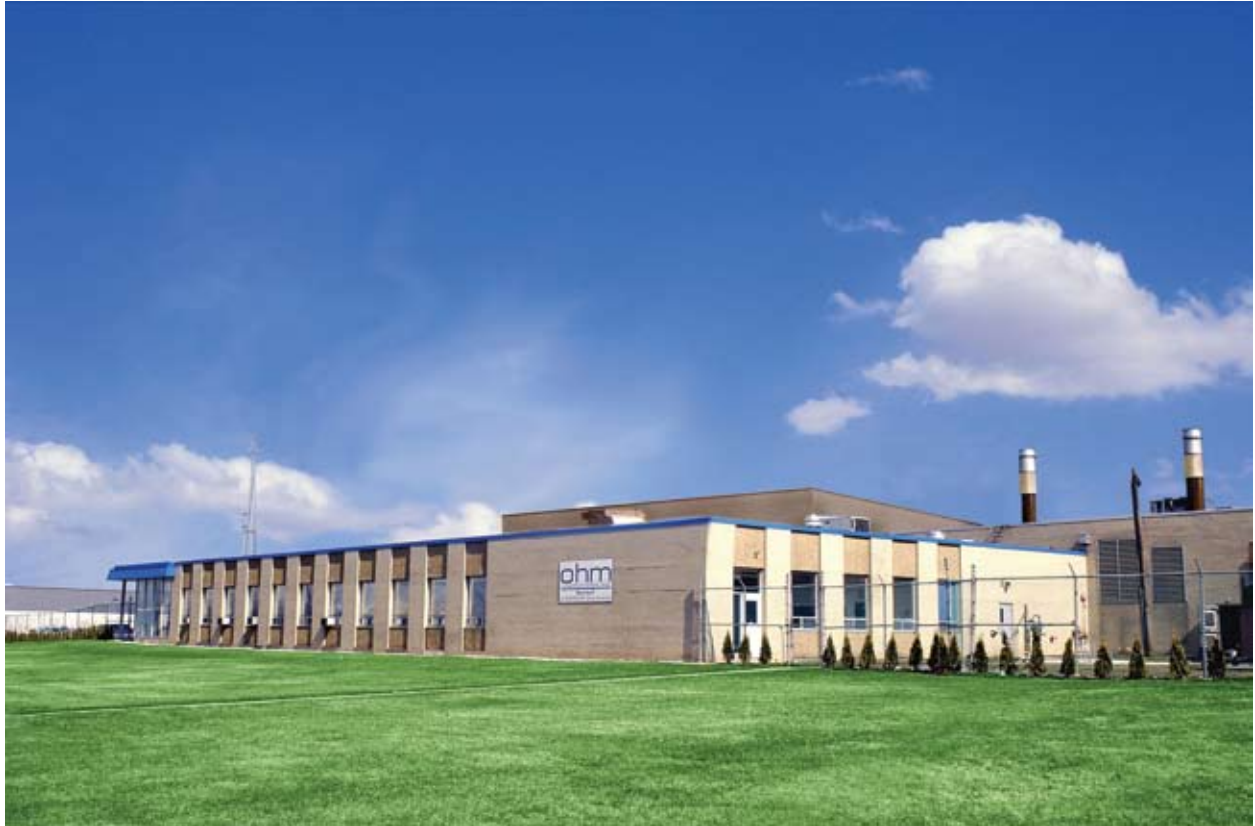
Ranbaxy Manufacturing Facility, New Brunswick, New Jersey
